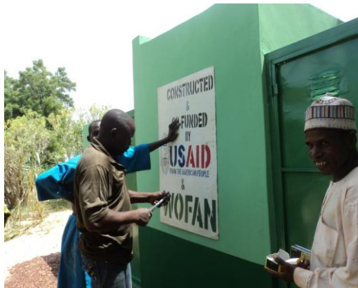
construction of urinals and Vip laterines in progress
